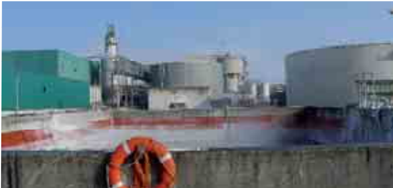
Sewage treatment water plant - Château-Thierry
